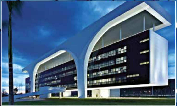
“CAMG” - Belo Horizonte, Brazil Project van Architect Oscar Niemeyer
